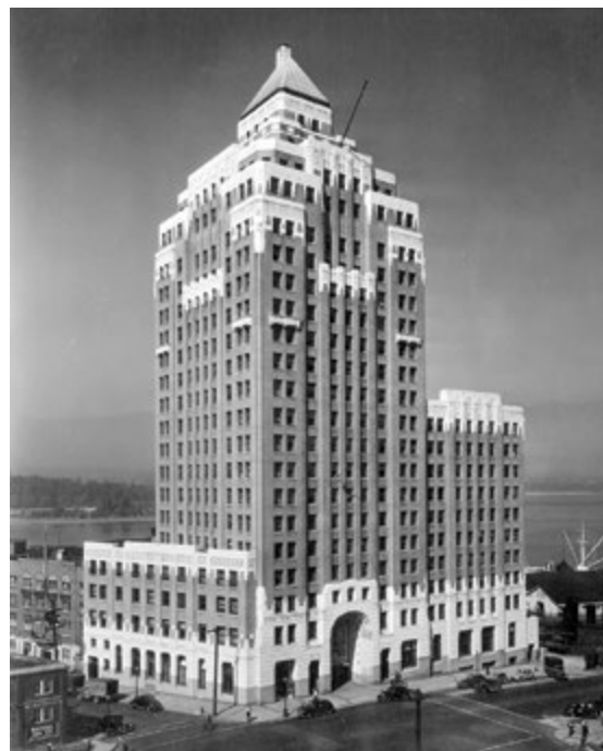
Marine Building in 1947
