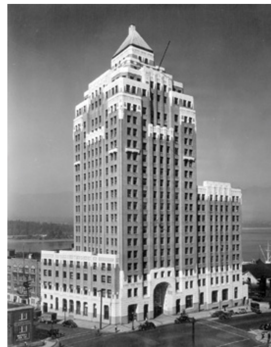
Marine Building in 1947
